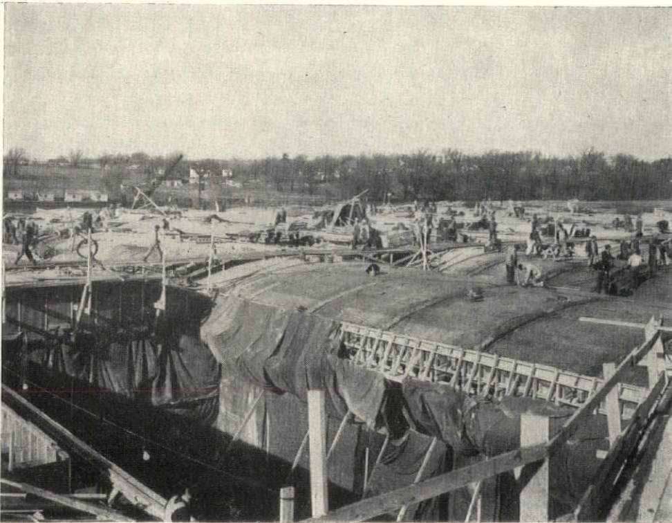
An "Orphan Bay," adjacent forms moved and ready for new setting.
