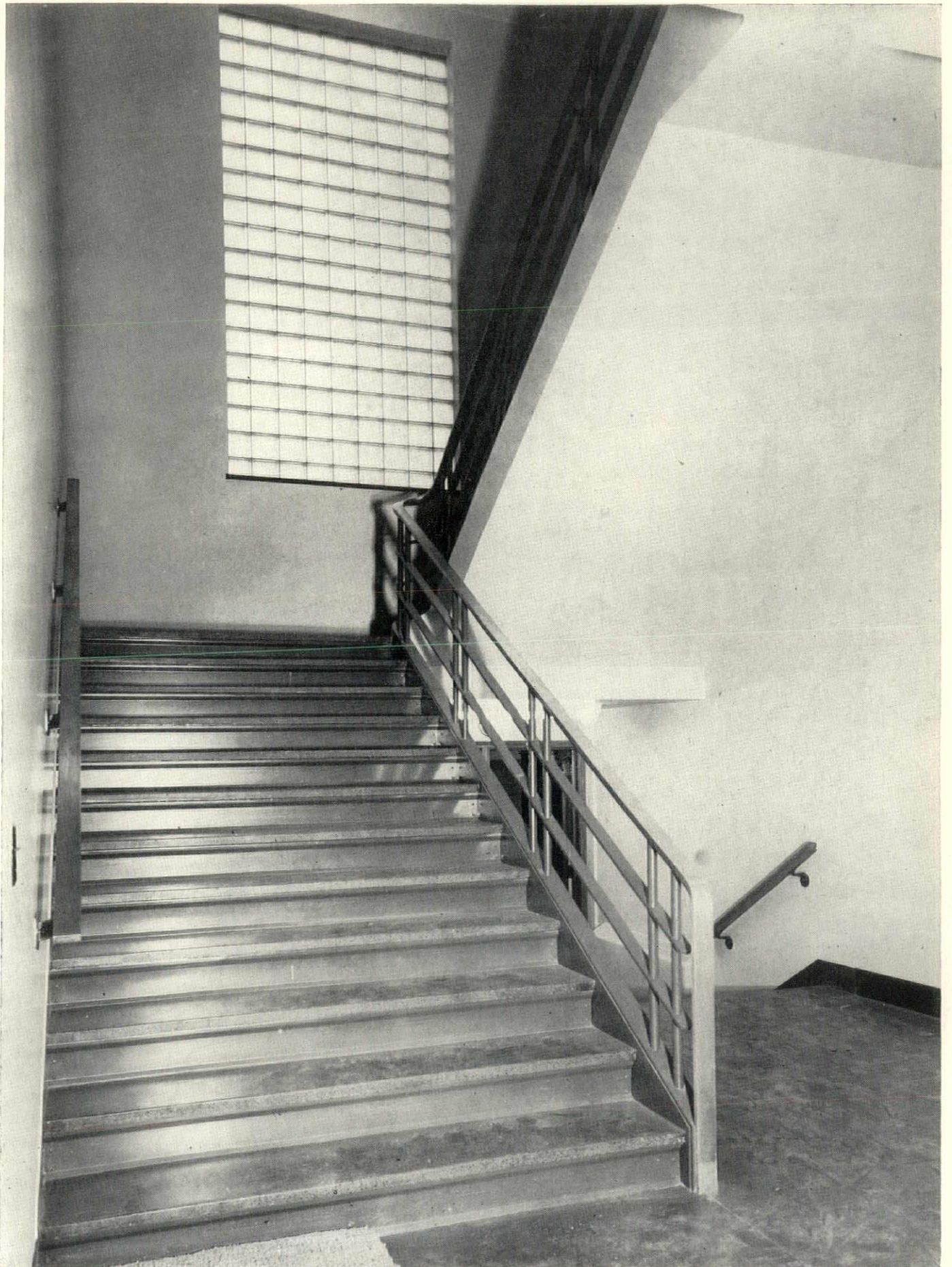
Main Stairway Office Building
