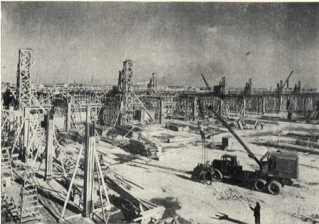
ENOUGH WOOD TO BUILD 2,000 FOUR-ROOM BUNGALOWS. Thirty million square feet (1,000 car loads) of lumber are being used for concrete forms and supports during construction at Chrysler Corporation's new Dodge Chicago Plant—to be the world's largest manufacturing unit. Recently it has been described as "big enough to put the Ford Willow Run bomber plant inside and have room enough to put 20 baseball diamonds around the edges."
