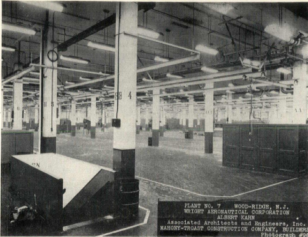
Columns are spaced 20 x 28 feet apart, and wide enough for a conveyor type of factory plan.
