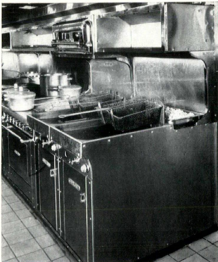
Gas-fired deep fat fryers in the gleaming modern kitchen of the Detroit Athletic Club.
