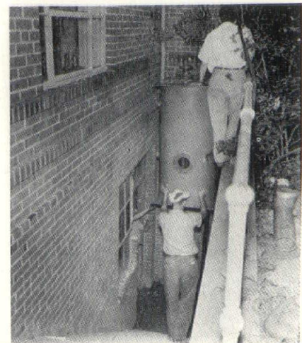
Rigging job made easy with "L-W" section
