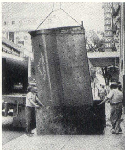
Rigging "L-W" boiler section through standard sidewalk access opening
