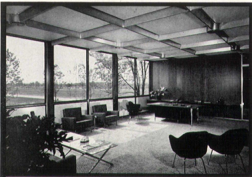
This executive office in the Research Administration Building shows a typical installation of Thermotank's custom-designed air diffusers with integrated sprinkler heads.
