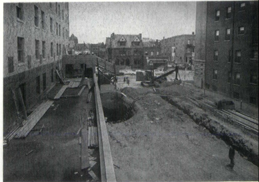
GARDEN SITE UNDER CONSTRUCTION
