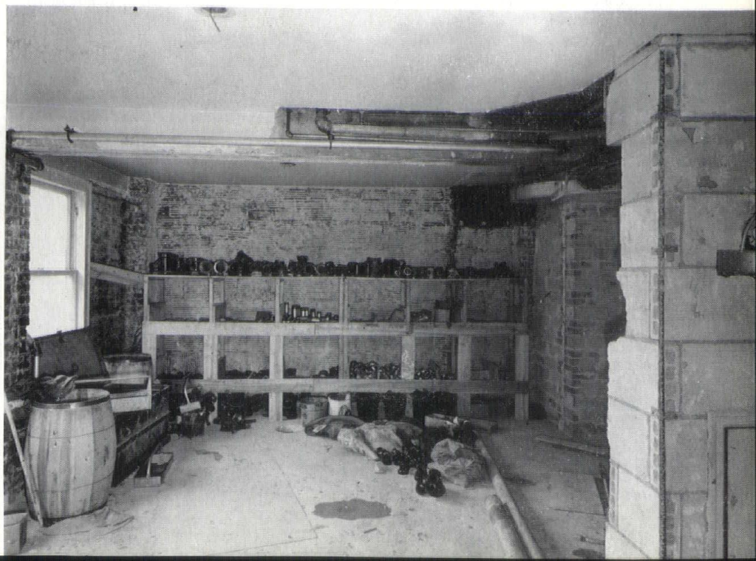
SUB-KITCHEN AREA BEFORE RECONSTRUCTION
