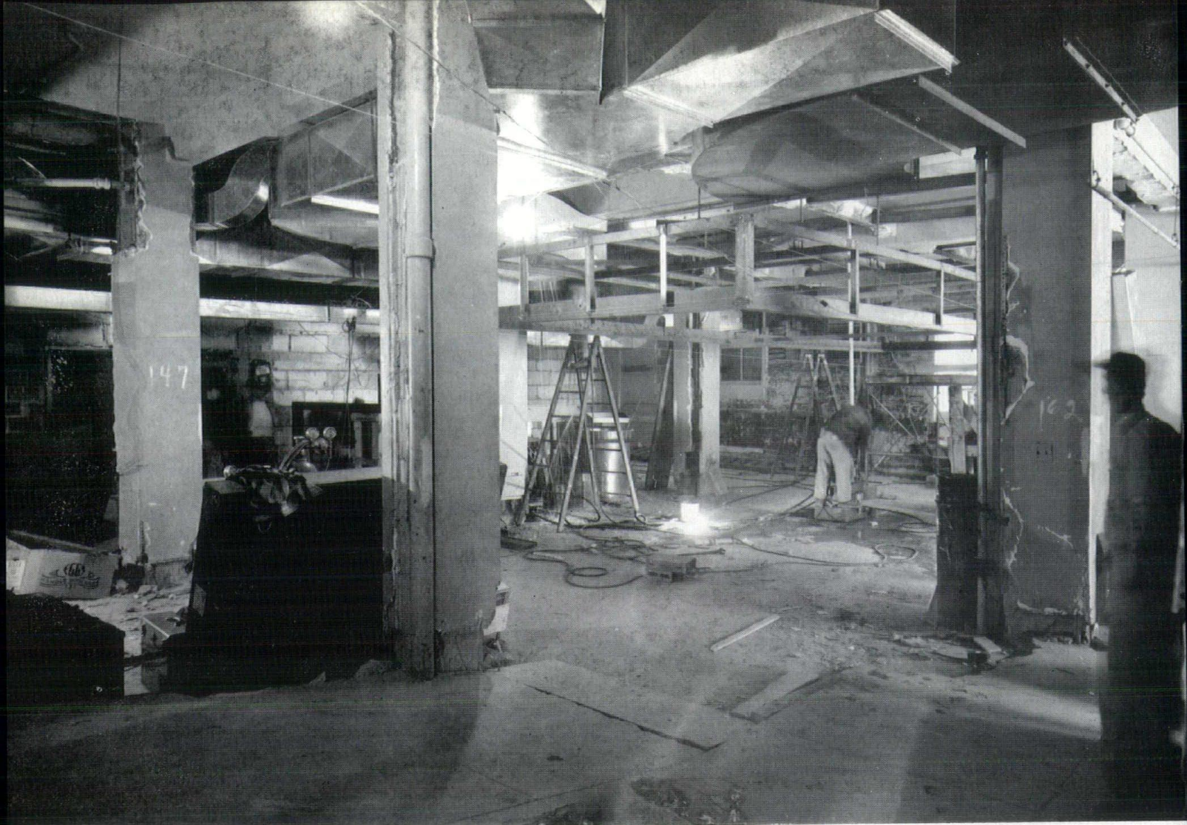
MAIN KITCHEN, FIRST FLOOR, BEFORE RECONSTRUCTION
