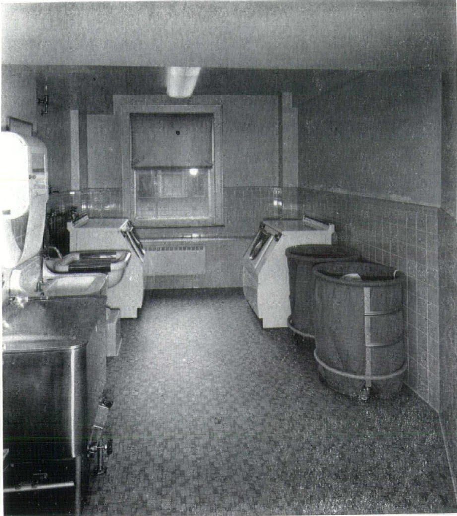
TYPICAL SOILED UTILITY ROOM INFIRMARY FLOORS
