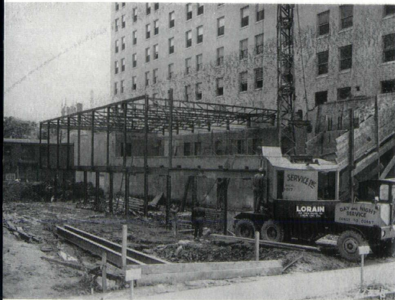
CHAPEL UNDER CONSTRUCTION
