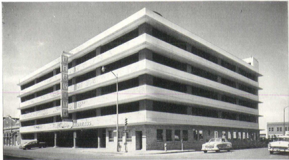
Knightley Parking Garage, Wichita, Kan. Architect: Overend & Boucher, Wichita
