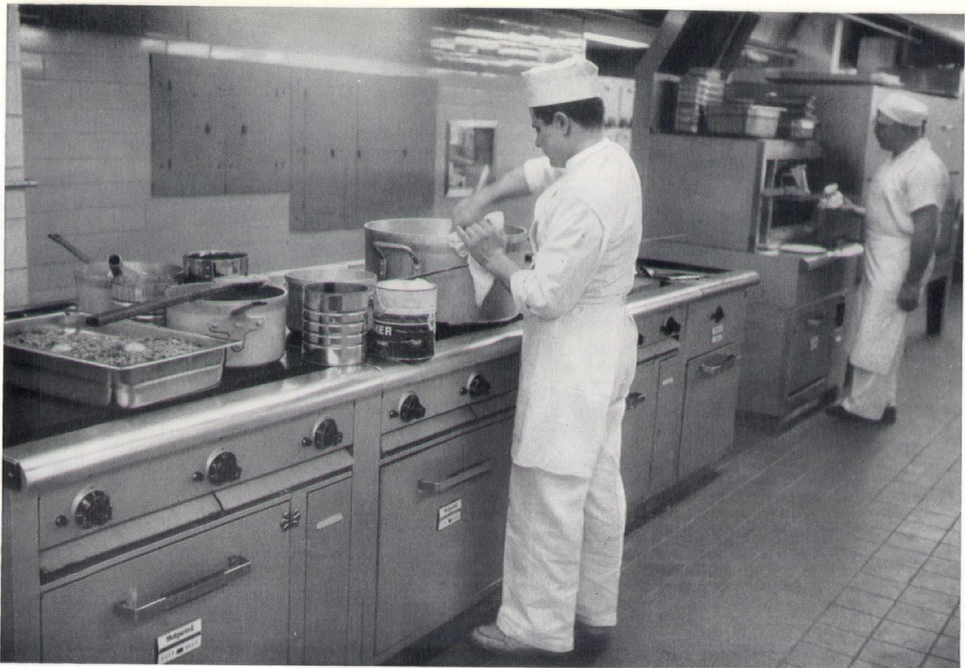
Electric range, deep fryer, broiler and bake oven are arranged for maximum efficiency in the all-electric kitchen of William Beaumont Hospital, Royal Oak.
