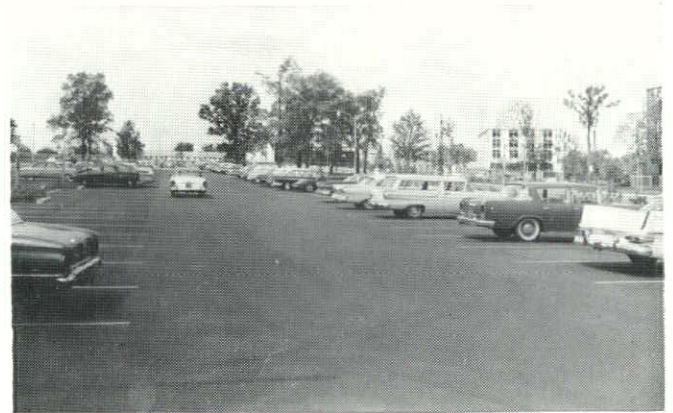
Asphalt Surfaced Parking Area
