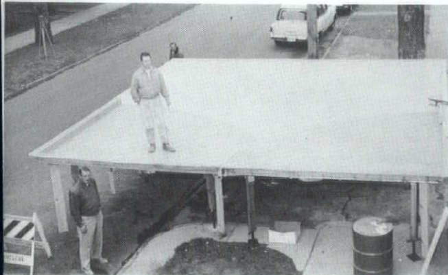
Plastic Form for Roof Slabs
