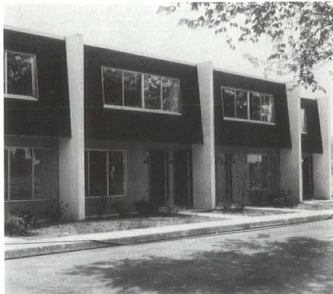
Nagel Plaza, a 24-unit complex featuring innovations in construction techniques suitable for low-cost housing, is situated a few blocks from areas ravaged during the Detroit riots of 1967.
