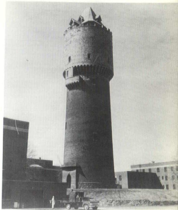
Kalamazoo State Hospital Water Tower
