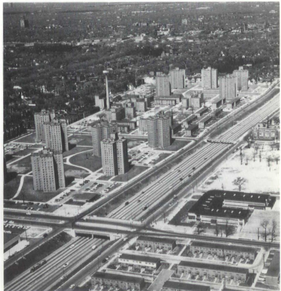
The Jeffries Project, overlooking the John Lodge Freeway in Detroit, is an example of the way that public housing has been built in the past. Harold Varner, Detroit Housing Commission Director-Secretary, says this kind of regimental living quarters is "a major indication of this country's continued relegation of the black and the poor to back corners of society. . . ." Varner has challenged architects and planners to show concern and take steps to change the concept of living quarters for the poor.
