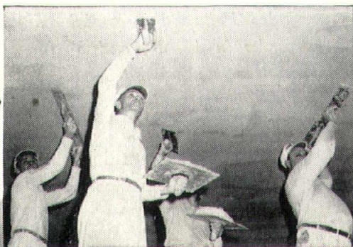
An attractive texture was obtained by stippling the ZONOLITE Acoustical Plastic.
