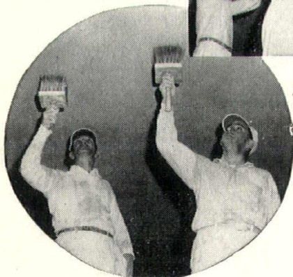
An attractive texture was obtained by stippling the ZONOLITE Acoustical Plastic.
