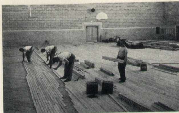
Laying the hardwood floor
