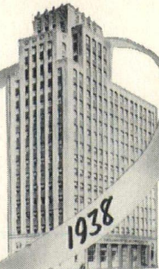
↑ Com'l Nat'l Bank, Shreveport, La.: Zonolite Plaster Fireproofing. The first use of Zonolite in Shreveport.
