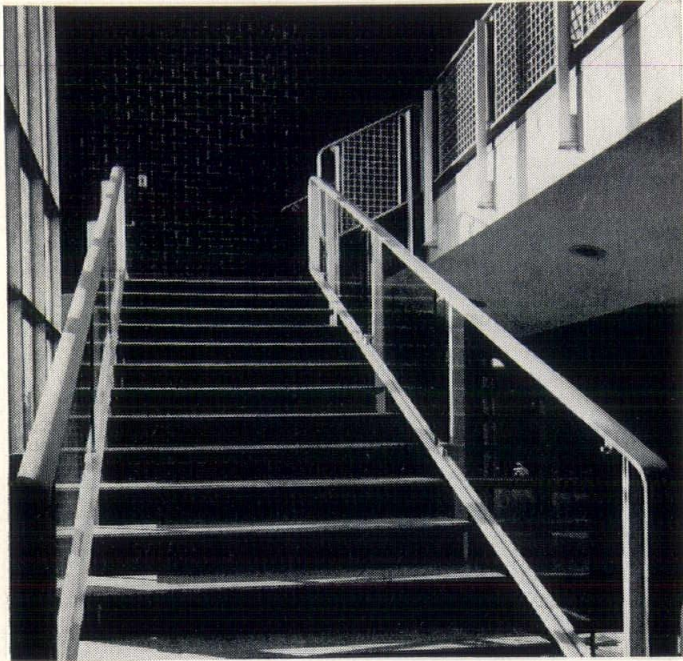
Closeup view of stairway showing the detail of railings and excellent metal craftsmanship in their fabrication.
