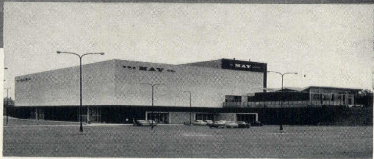
Single and Twin-Arm Millerbernd standards light the 2,000-car parking lots and the approaches to this ultra-modern suburban department store. Millerbernd High-Strength steel construction with heavy tapered bases can take the punishment of parking lot services.
