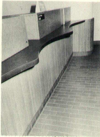
Quarry Tile flooring and Black Slate check desk and ledges. All furnished and installed by
