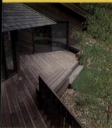
Air Dried Construction Common; Builder: Robert H. Mason, Inc.; Location: Minnetonka, Minnesota
