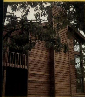
Ruf Rider 10" Super Thick Butt Redwood Bevel Siding; Builder: Cramer-Weir Company; Location: Bloomington, Minnesota
