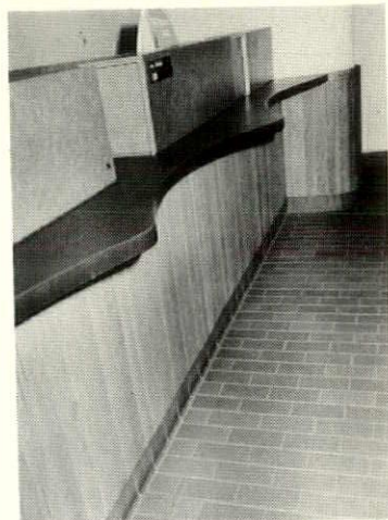
Quarry Tile flooring and Black Slate check desk and ledges. All furnished and installed by
