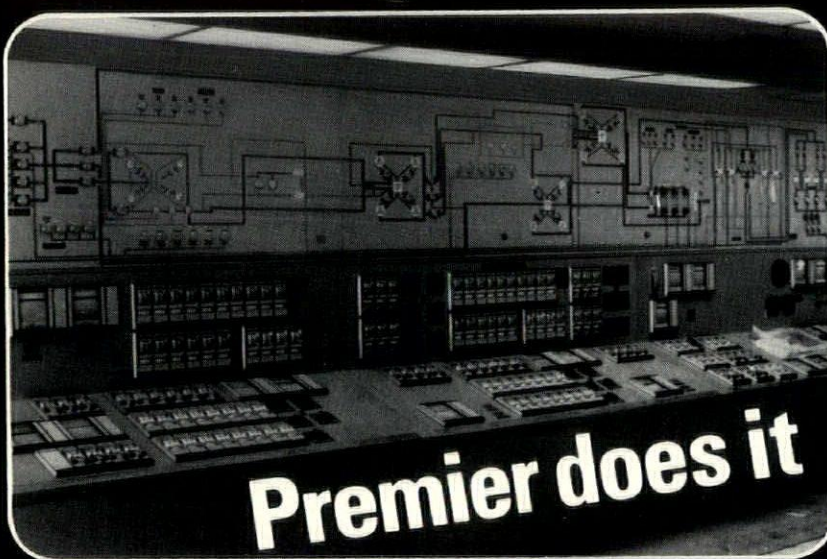
Master control panel at Salt Creek Sewage Treatment Plant.
