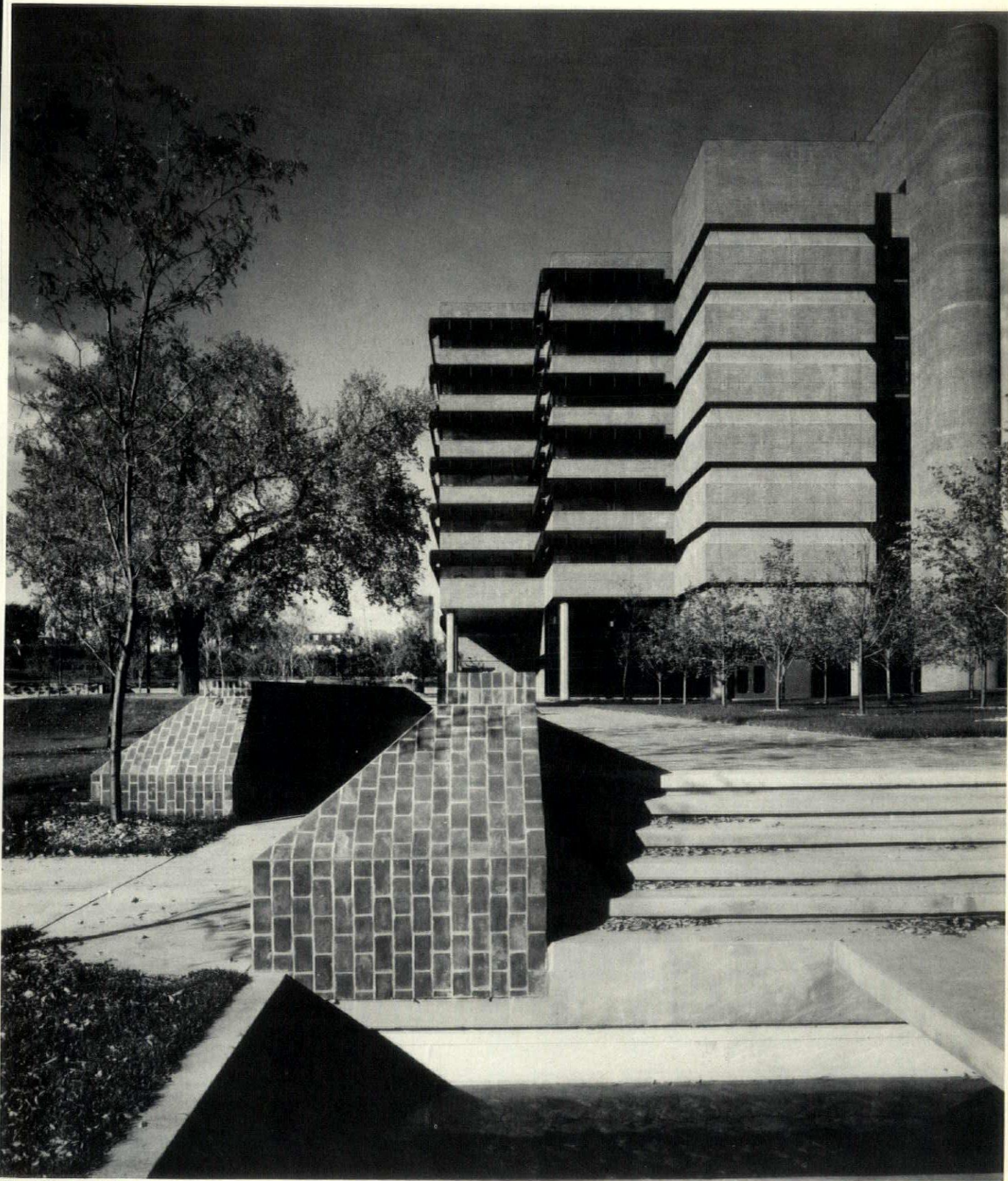
Plaza West building
