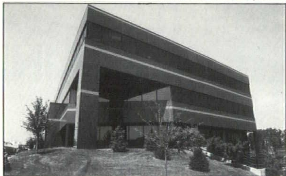
CENTRE POINTE ONE, MENDOTA HEIGHTS, MN GLAZING CONTRACTOR—EMPIREHOUSE, INC.
