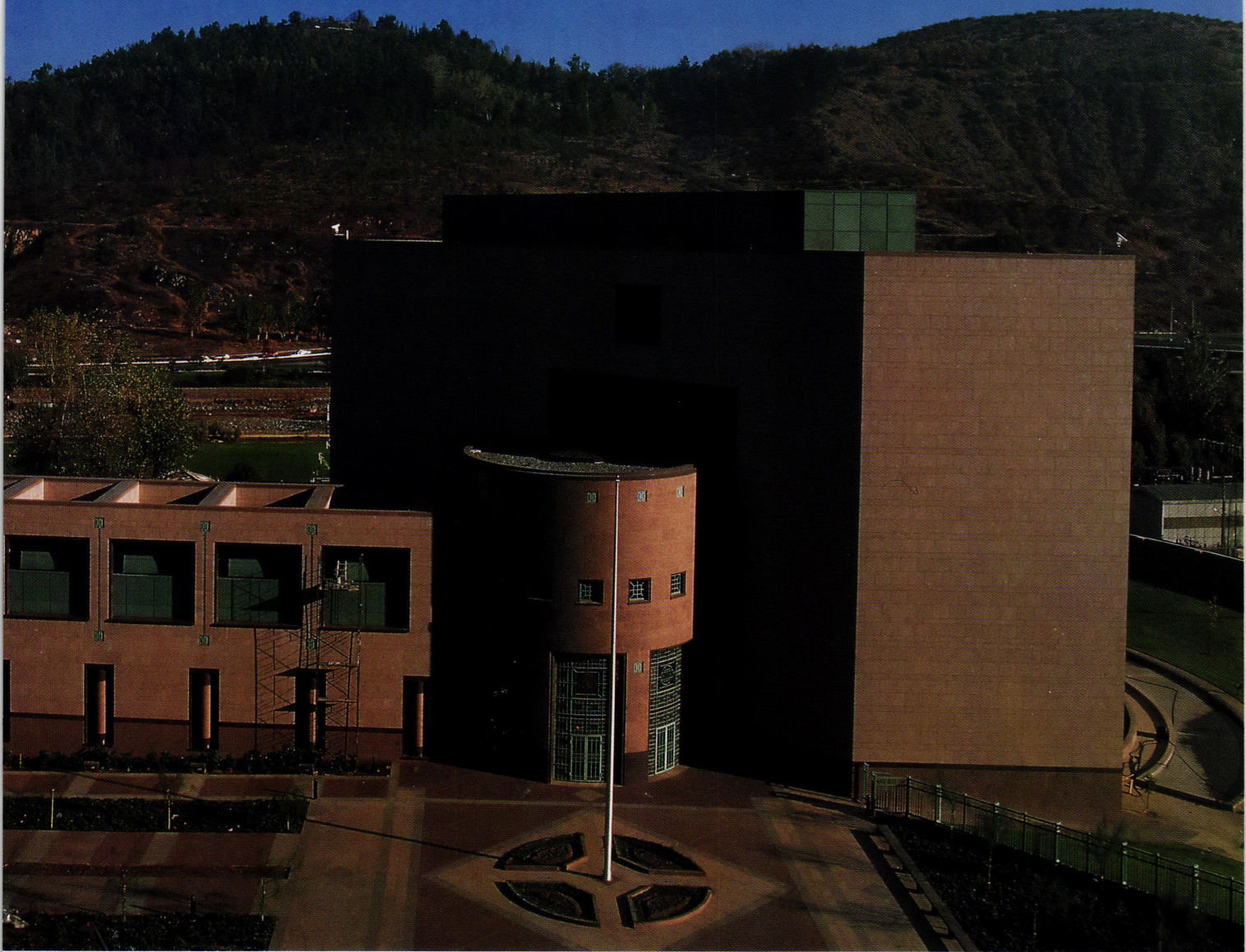
The U.S. Embassy, built to withstand terrorist attacks, is divided between publicly accessible functions in a 2-story, rectangular wing (above) and secure embassy functions in a 5-story midrise (left). A diagonal, slab-like structure symbolically divides public from private. An arbor (opposite left) connects with the extensively landscaped grounds.
