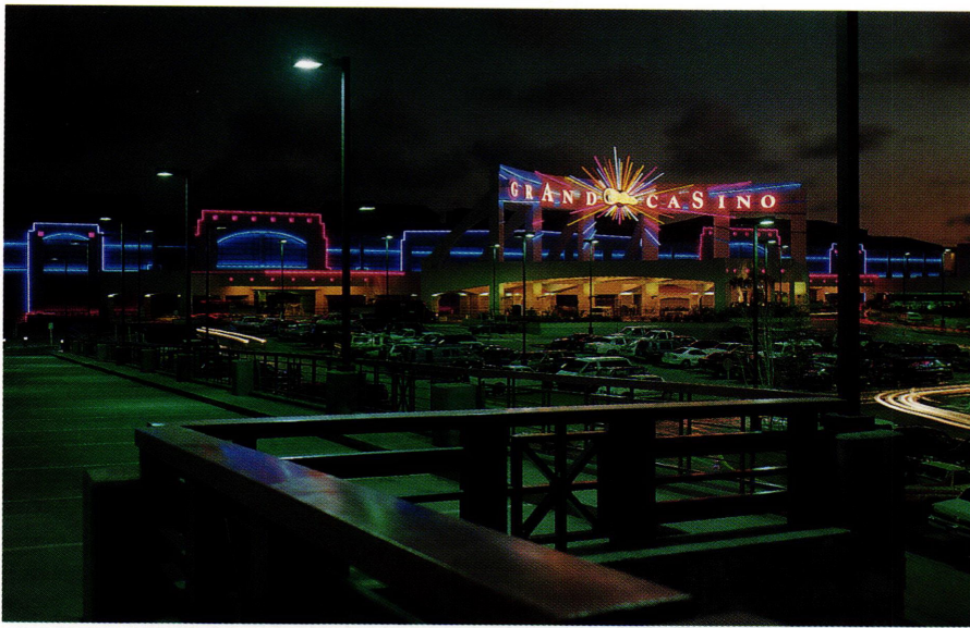
A curving glass wall opens the theater (bottom) to the busy street. The theater's lobby (below), functional if not particularly luxurious, acts as a large circulation corridor that moves patrons quickly between the casino and theater. Colorful lights call attention to the floating casino (left) at night.
