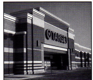
The Target Store in Sillwater, Minnesota, illustrates the smart look of 4" high decorative rock face CMU's complemented by 4" and 8" high Ground Stone Masonry Units to provide the ideal combination of strength, aesthetics and economy.
