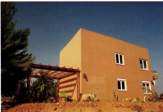
A rooftop deck (top) overlooks the sea. The house is composed of two geometric forms (above), which burst open on the sea-facing side (opposite top). White plaster walls and tile floors (opposite bottom) enhance the interior.
