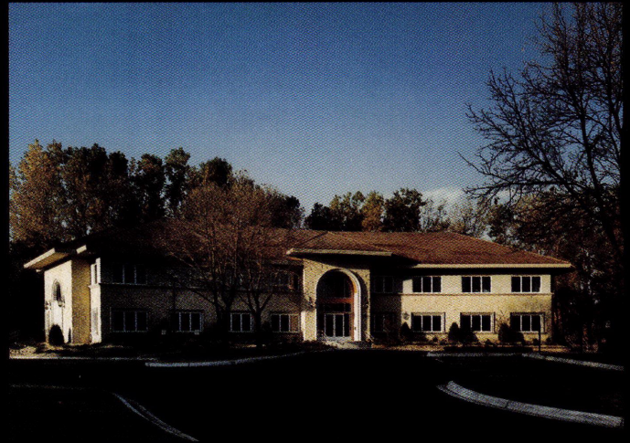
Minnetonka Office Building
