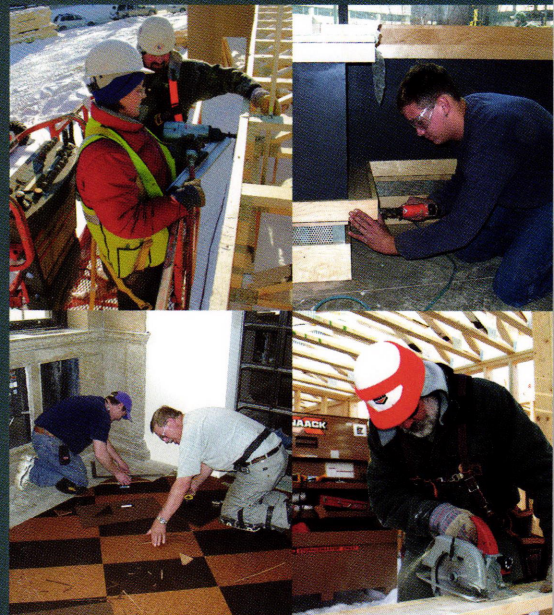
construction photographs by Jeffrey Miller
