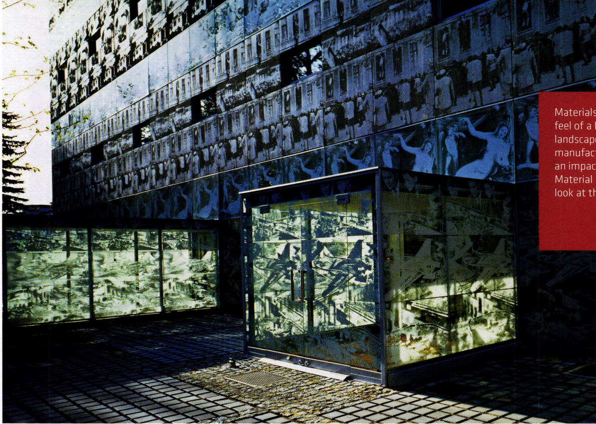
Herzog & de Meuron used a photoengraving technique to animate the bands of concrete panels that wrap the Eberswalde Technical School Library in Germany (above). The LiTraCon company markets translucent concrete blocks cast with optical glass fibers (right). These and other innovations are changing perceptions about concrete.
