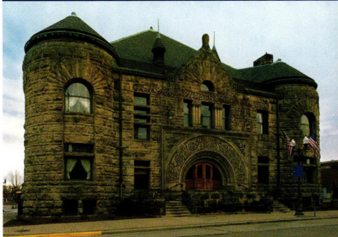
The Richardsonian south façade of the 1889 Mabel Tainter Memorial Theater in Menomonie, Wisconsin.
