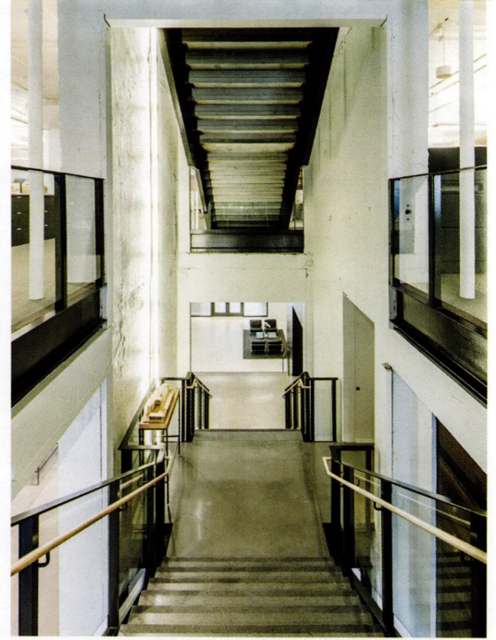
In HGA's hands, the Ford Center's original Model T showroom became a dramatic reception and gallery space with a row of flexible meeting rooms. The central staircase sits in the old elevator shaft that used to carry cars down the plant's vertical assembly line.
