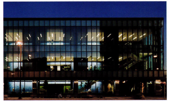
MCTC Health Sciences Renovation
