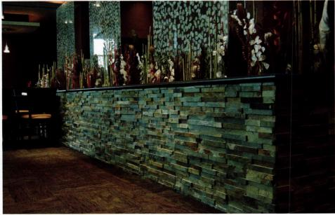
Realstone System panels are made of authentic split stone - slate, quartzite or sandstone — cut and formed into panels for exterior or interior applications. Realstone System panels join together seamlessly. Corner pieces are cut with fingered ends joining each panel together with strength and without visible seams. Realstone System panels are available in multiple colors and textures. They revolutionize the installation of natural stone, reducing cost, weight and installation time.
