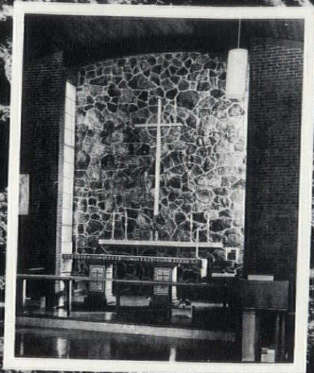
St. Stephens Episcopal Church — St. Louis Charles Novak Jr., Architect
