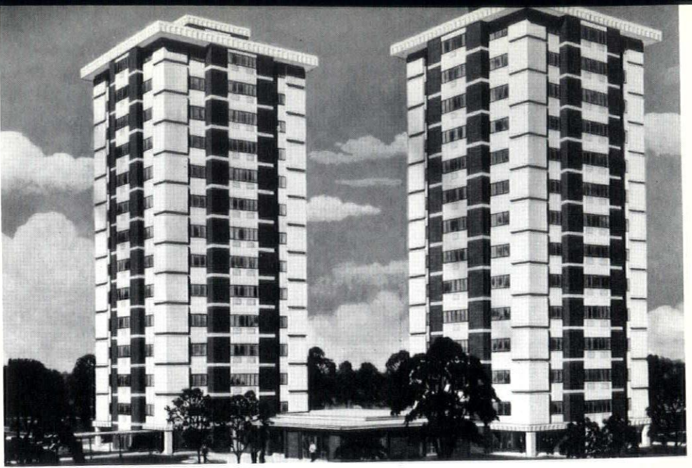
Twin tower high-rise, Poplar Bluff, was designed by Butler and Associates for elderly, low rent occupancy, will house 264 families. Special features include private kitchen facilities, convenient laundry facilities, adjoining community center and recreation areas.
