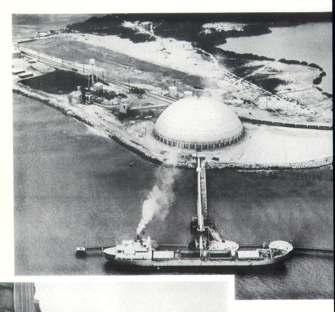
A new Caribbean landmark is Alcoa's huge aluminum dome bauxite storage shed at Rocky Point, Jamaica. Bauxite comes from mines in 86-ton aluminum rail cars (right). From an open storage area (dark patch, top left), ore is screened, dried, and moved to the dome to be kept dry until loaded aboard ore carriers.
