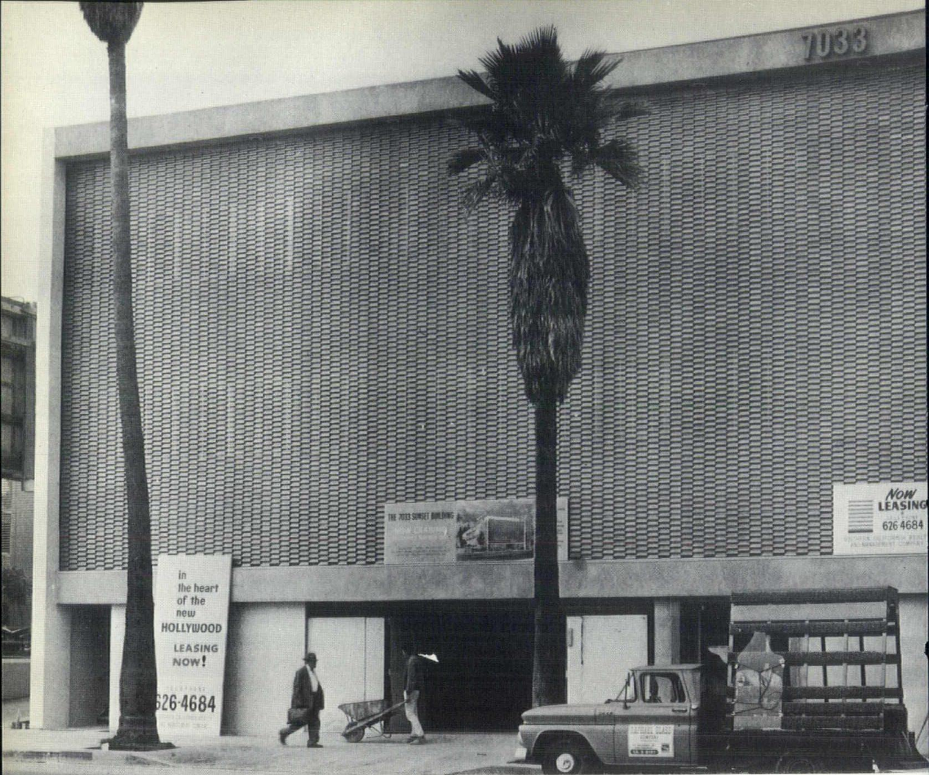
LIMITED HEIGHT building at 7033 Sunset Boulevard, Hollywood, receives finishing touches to put it into condition for occupancy by many tenants who execute leases during the construction period. Designed by Irving D. Shapiro, A.I.A., the building features second-story reflection pool patio area and ground level parking.
