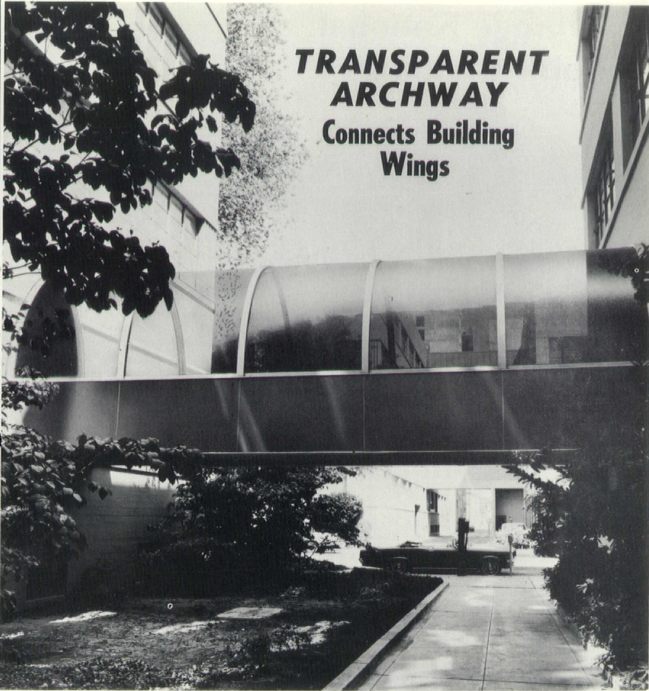
Employees in Sacramento's Public Works Building easily go from one wing to another via this 30' long transparent bridge. Made of gray tinted Plexiglas acrylic plastic, the transparent enclosure is weather-resistant and resists breakage from impact.
