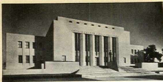
Iberia Parish Court Building in Louisiana was designed in architectural concrete by Architect A. Hays Town of Baton Rouge
