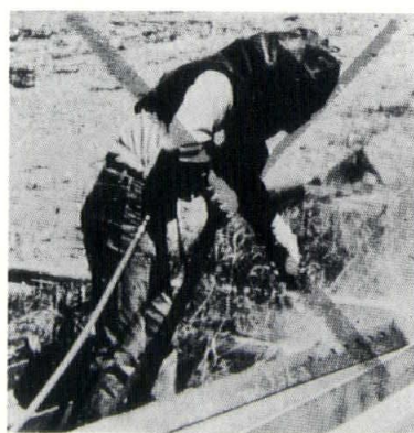
Obsolete— Manual Sand Blasting— More Costly, and Shop Health Hazards!
