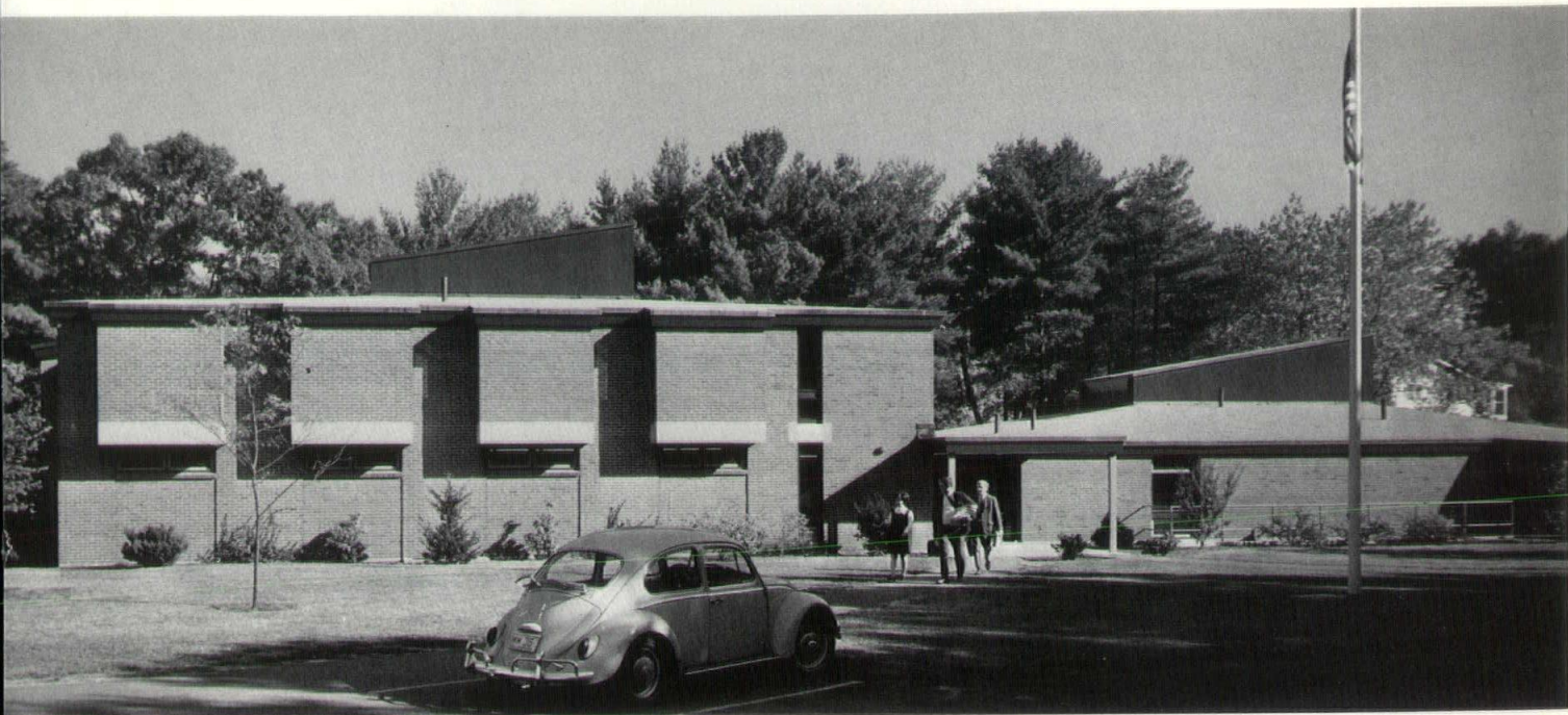
The west side; the slanting structures are skylights.
