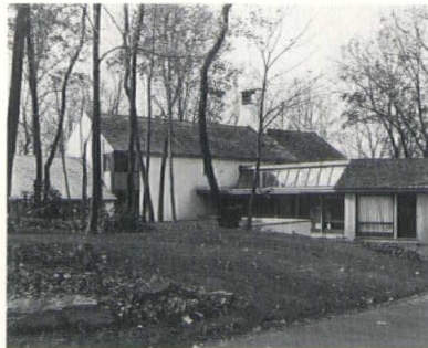
Residence, Princeton Township
