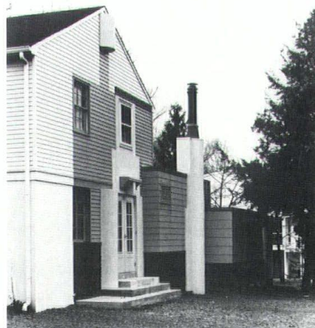
Schulman House Addition
