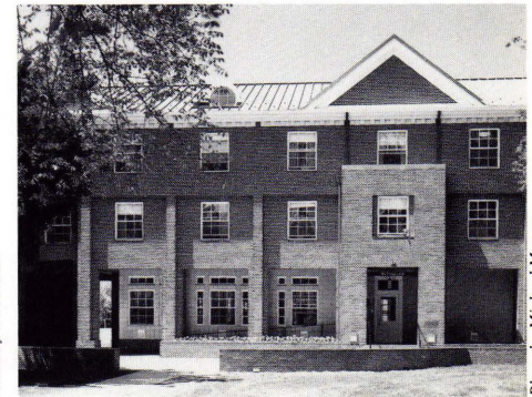
Reynolds House Dormitory, Lawrenceville School
