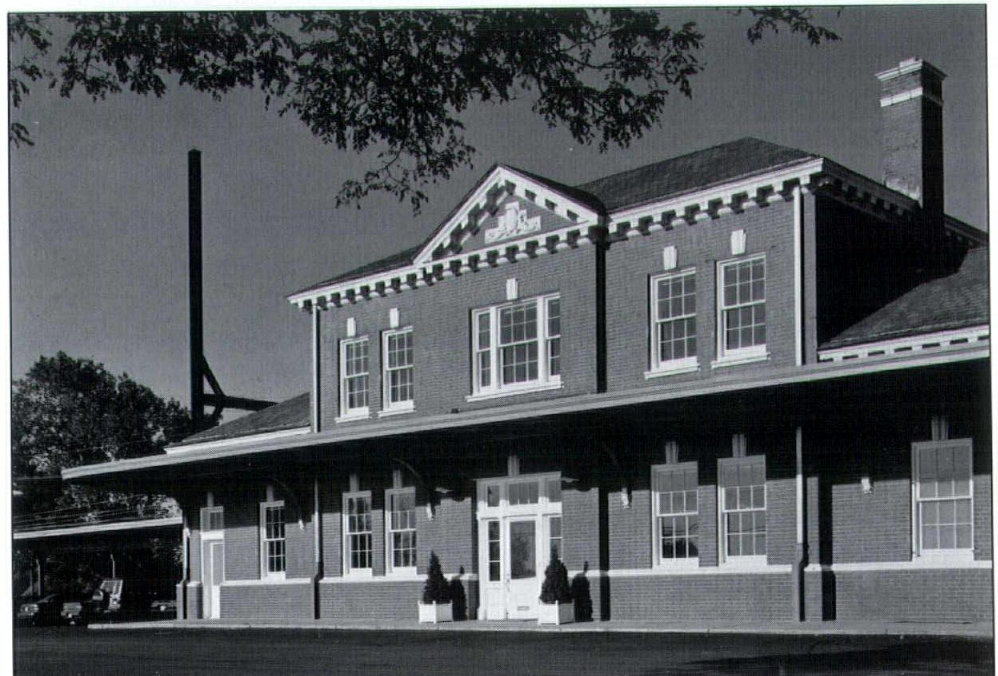
Restored street facade.
