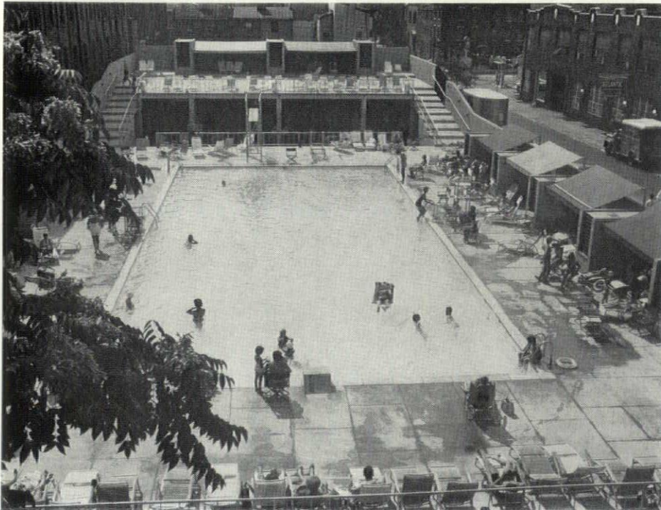
1. Rittenhouse Swim Club. Built out of concrete block and pre-cast concrete in one continuous piece, buildings, pool and decks are all integral.
