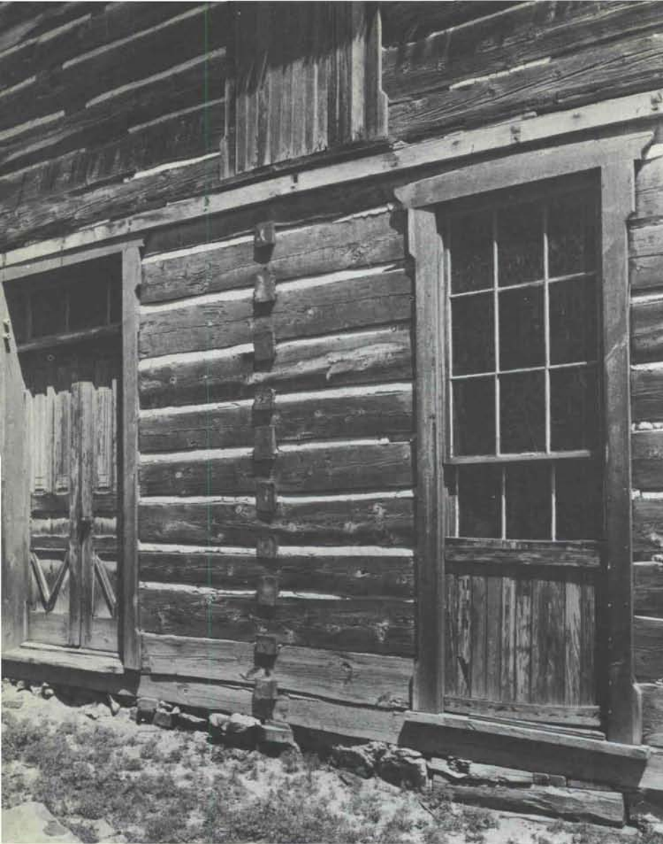
The elegance of front door and window details, and the superbly joined hand hewn beams of the formal log portion.
