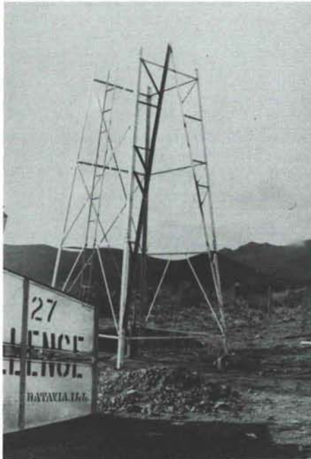
Building a steel tower up one piece at a time in the Guadalupe Mountains of New Mexico/Texas in the 1930's. Photograph courtesy B. H. Burdick, Sr., and Panhandle-Plains Historical Museum, Canyon, Texas.
