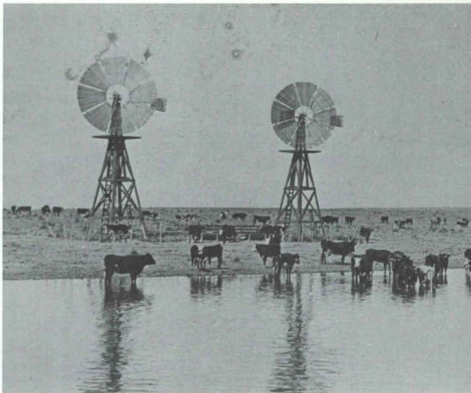
Two "Railroad Eclipse" windmills on telescoped wooden towers at Twin Wells in eastern New Mexico early in this century. Courtesy Garnet Brooks, Shamrock, Texas.
