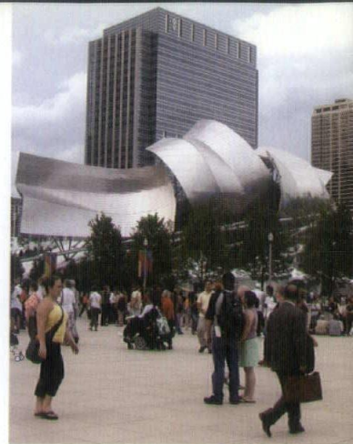
Other Gehry icons (clockwise, from left): Prague's Dancing Building, Chicago's Pritzker Pavilion and LA's Disney Hall.
