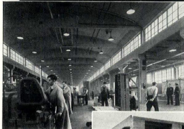
Interior of war industrial plant having 38 and 60-ft. bays spanned by ribbed concrete arch roof. Albert Kahn Associated Architects & Engineers, Inc. Geo. A Fuller Const. Co., contractor. (Photo courtesy Dodge Chicago Plant, Division Chrysler Corp.)
