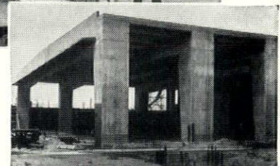
Hollow, reinforced concrete rigid frames have 150-ft. clear spans in twin National Guard hangars at Des Moines, Iowa. Architect and Engineer, Wm. N. Nielsen; Structural Engineer, Les Forsyth; both of Des Moines.
