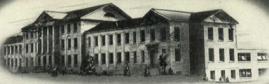
ENGINEERING BUILDING UNIVERSITY OF BUFFALO
