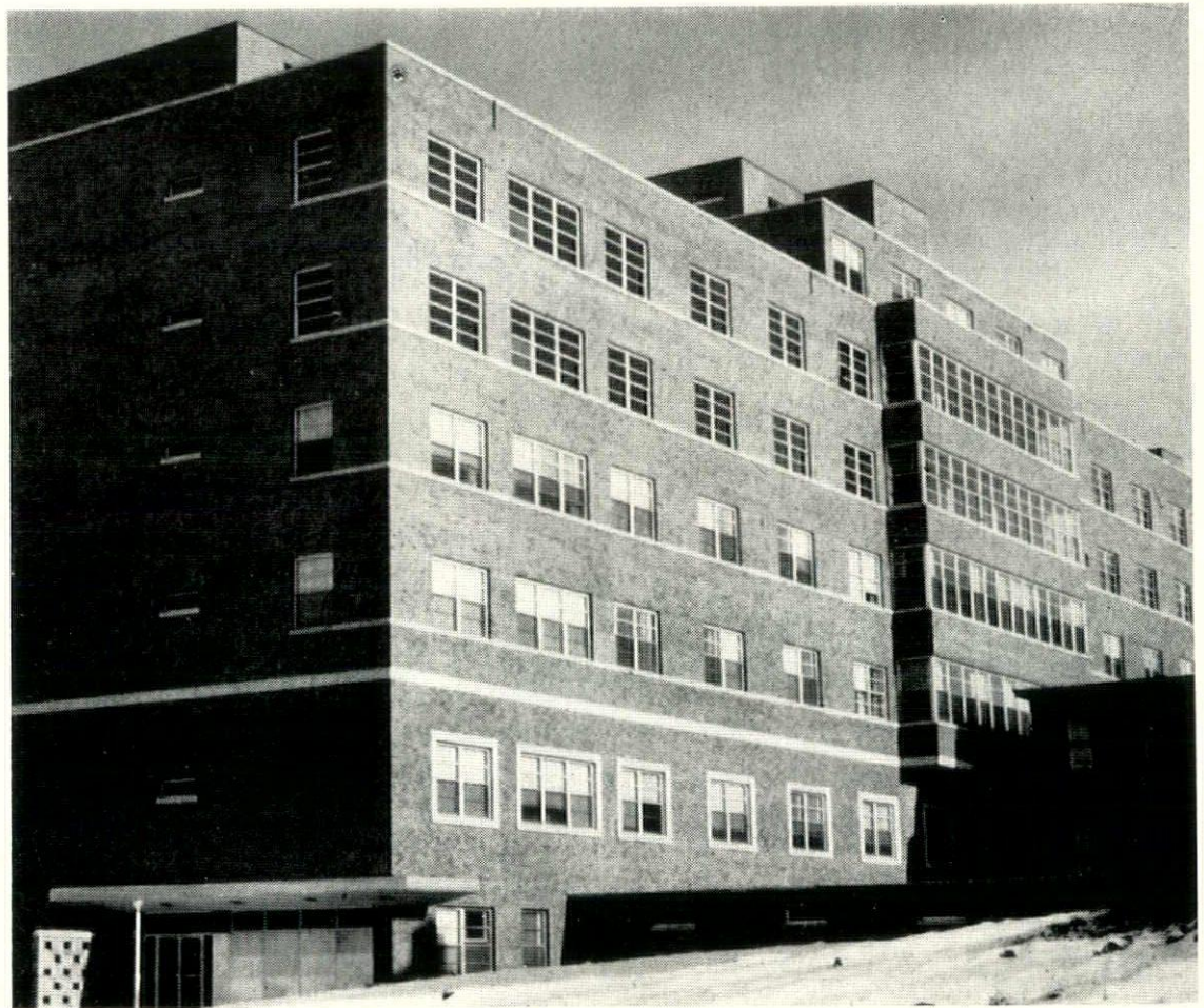
THE GENESEE HOSPITAL, ROCHESTER, N. Y.
