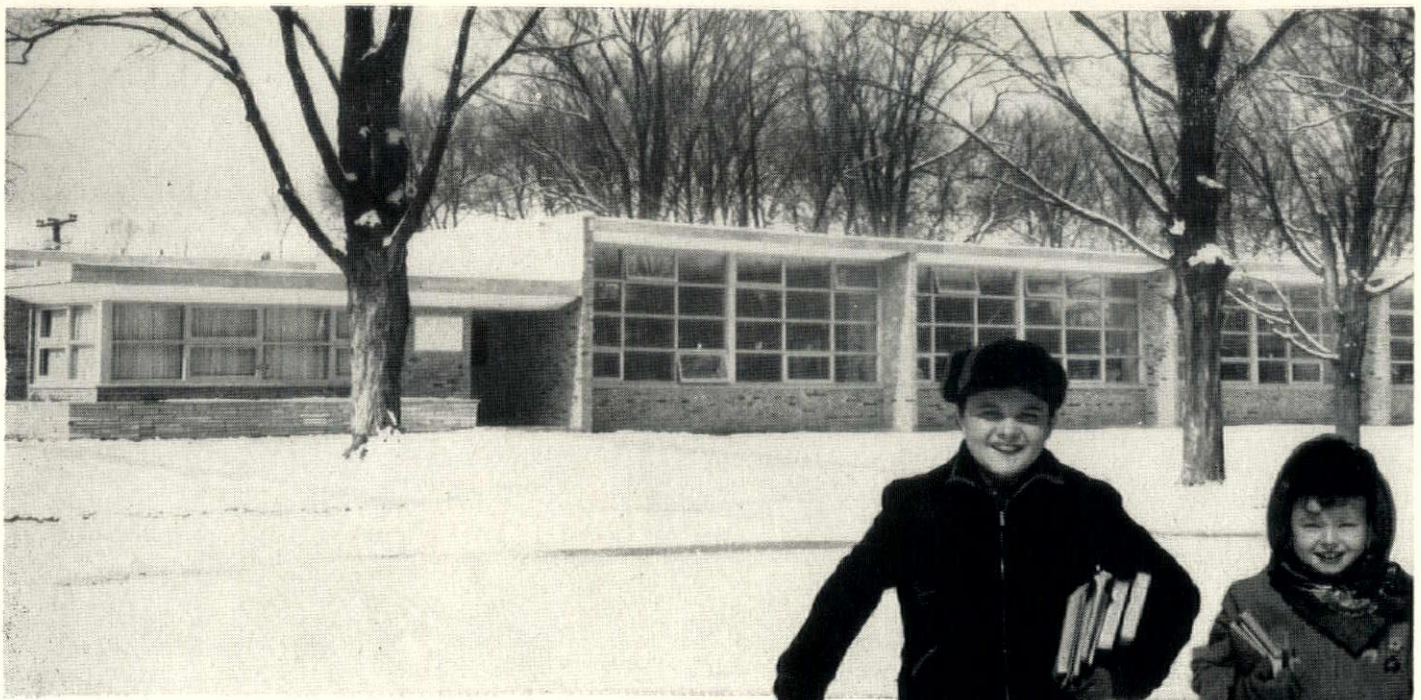
Daylight Walls of Thermopane insulating glass provide light, view and comfort for children in St. Patrick's School, Brighton, Mich. Architect, Charles D. Hannan, Farmington, Mich.
