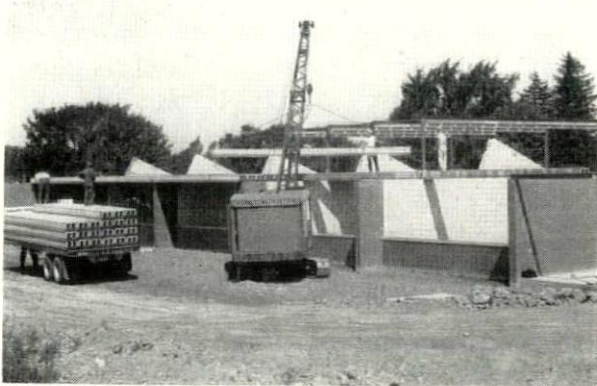
Two-way cantilevers. Self-supporting and inexpensively accomplished. Town of Tonawanda Building.
