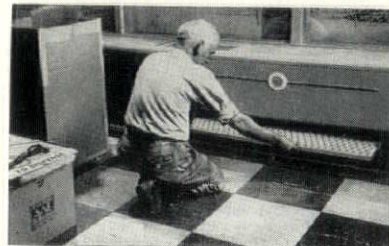
Replace filter in unit ventilator.
