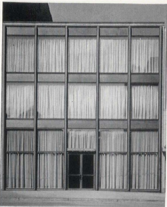
Northeastern Pennsylvania National Bank and Trust Co., Scranton, Pennsylvania. The bronze front of this building characterizes modern design employing extruded shapes of Architectural Bronze and sheets of heavy-gage Muntz Metal. The two materials are combined with glass to provide the enduring beauty and feeling of stability so important in banking institutions. All of the bronze was treated to produce a statuary bronze finish. Architect: George M. D. Lewis, Scranton. Fabricator: Standard Iron Works, Scranton.
