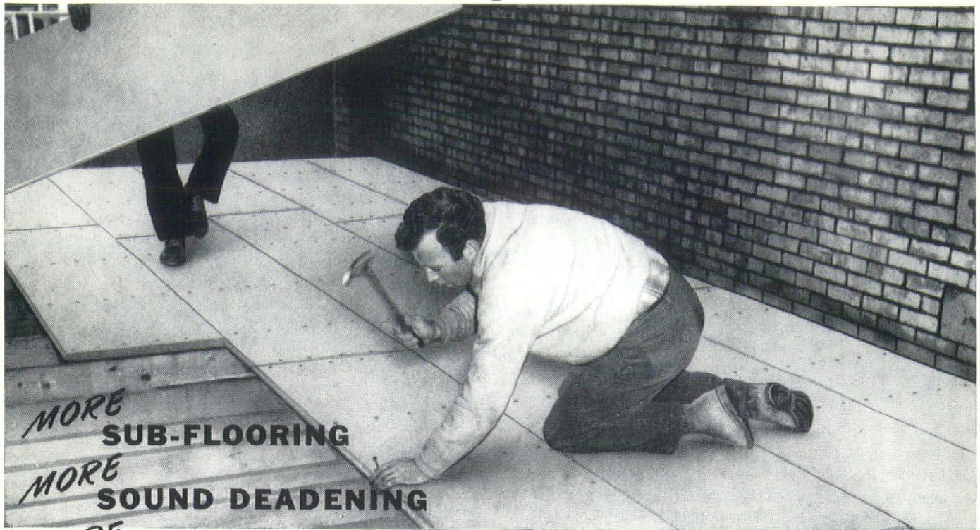
Installation of Homasote "4-Way" Floor Decking at Pickwick Motor Inn, Plainview, N. Y. Architects: Samuel Paul, A.I.A. and Seymour Jarmul, A.I.A.
