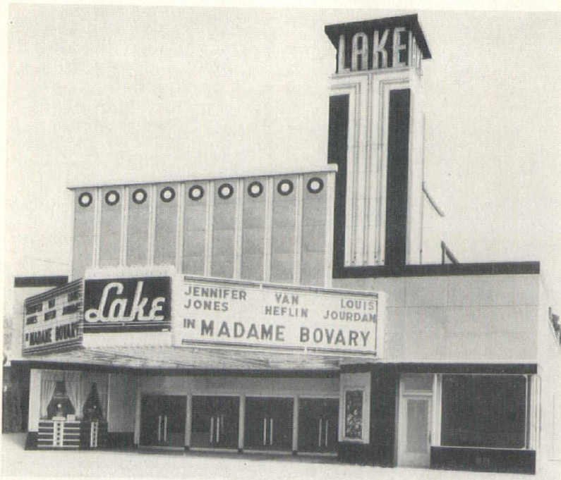
LAKE THEATRE — E. 226th St. and Lake Shore Blvd. Paul Matzinger and R. J. Grosol, Architects
