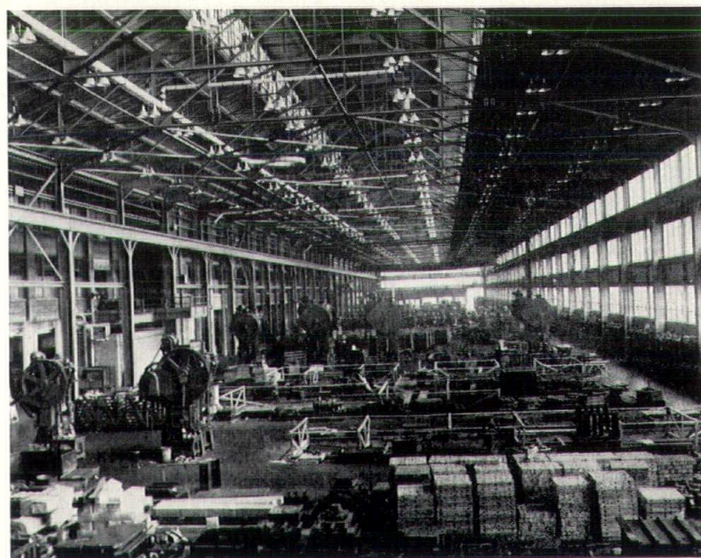
Interior of Perfection's Ivanhoe Press Building, Looking east.
