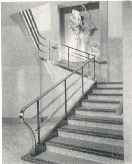
Stainless Steel Stair Railing and Stringer Cover for The Halle Bros. Co. Euclid-Huron Building, Cleveland. Architects: Walker & Weeks. General Contractor: The Sam W. Emerson Co.
