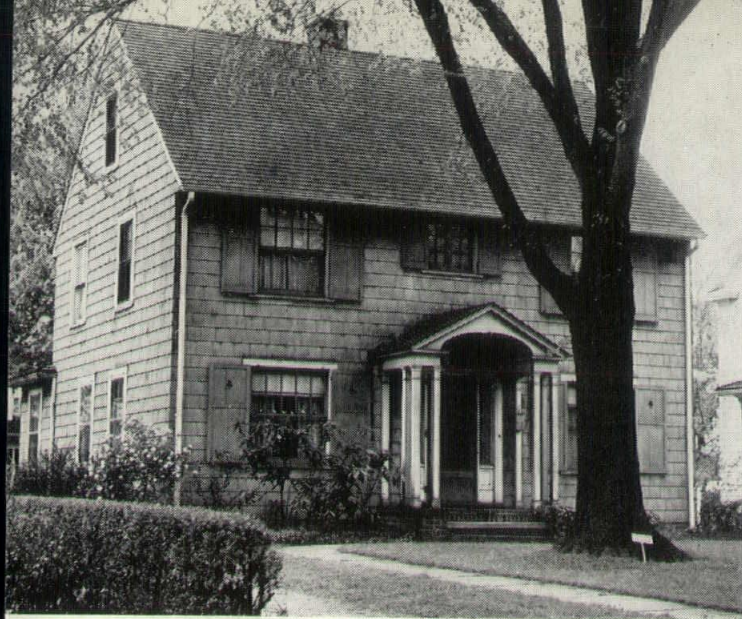
This house is typical of thousands more in this area. Built during the 1920 building boom, it is still structurally sound. All it needed was renovation and revitalizing.
