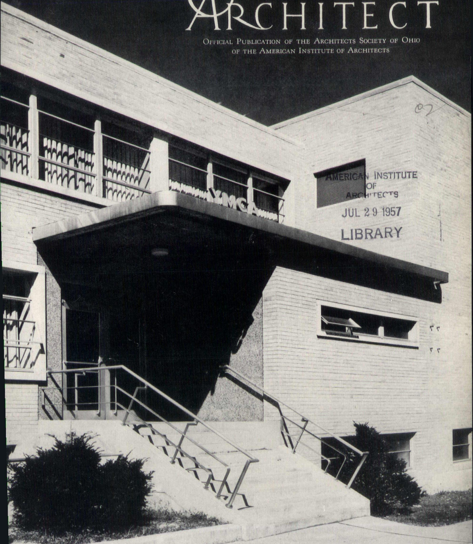
Northeastern Y.M.C.A. - Y.W.C.A. Main Entrance
