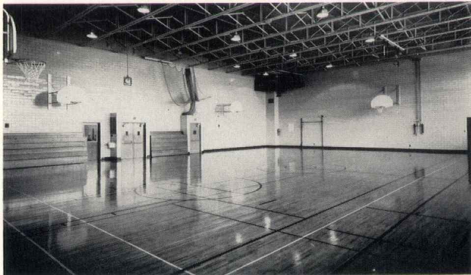
View of the Northeastern YMCA-YWCA gymnasium
